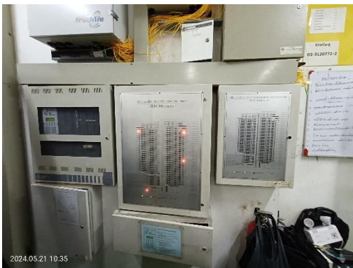
Fire Alarm Control Panel
